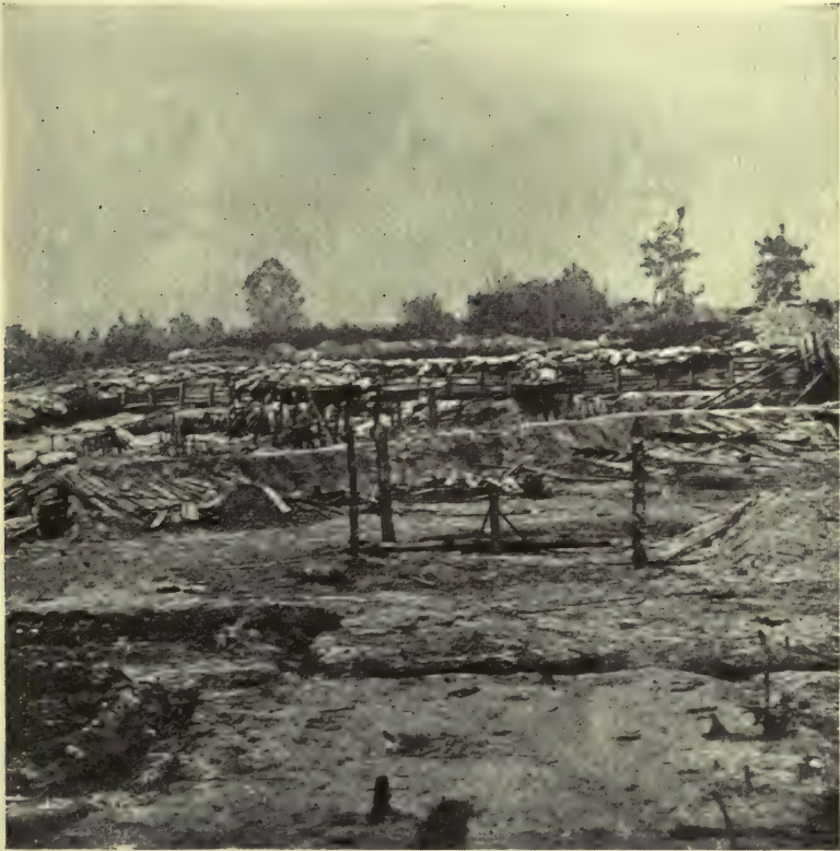
WORKS AT PRIEST CAP, PORT HUDSON
